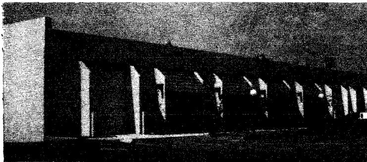
NEW G.A.S. CO. 20,000-SQ. FT. PRODUCTION FACILITIES.
